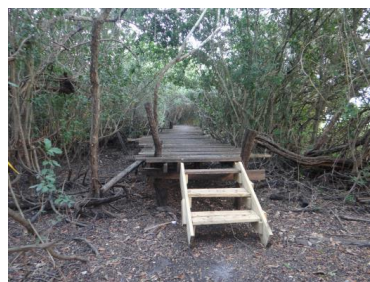
Figure 60. Elevated Walkway Over Areas that Flood in the Wet Season.
